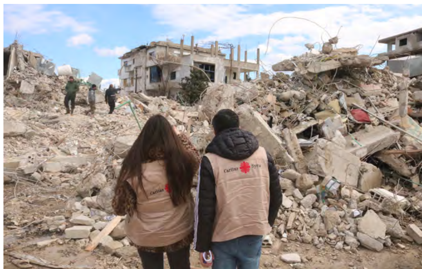
Caritas staff survey the destruction caused by the devastating 7.8 magnitude earthquake that struck northwest Syria and central Turkey on February 6, 2023. Photo courtesy of Caritas Syria.
